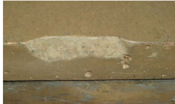
This same area is softened up by hand sanding it with 100 grit sandpaper. It should be re-sealed (not shown), to protect it and help it match the rest of the countertop.
